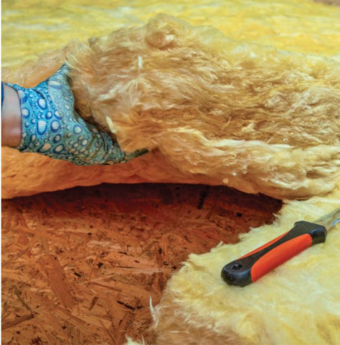
**Room in Roof Insulation** - By employing the latest insulation materials and methods, insulating existing attic rooms means that you can still use the roof space for storage or additional room space if needed while still trapping heat in the property and rooms below. A room in roof or attic room is simply defined by the presence of a fixed staircase to access the room.
